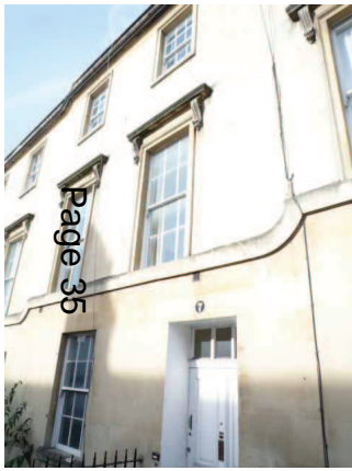
E) Refurbishment and extension of a Grade II listed building incorporating energy conservation measures (7 Charlotte Street; view application)
