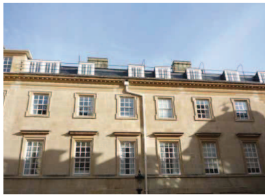
A) New slim-profile double-glazed windows in Grade I listed building (St John's Hospital, Bath City Centre; view application)
